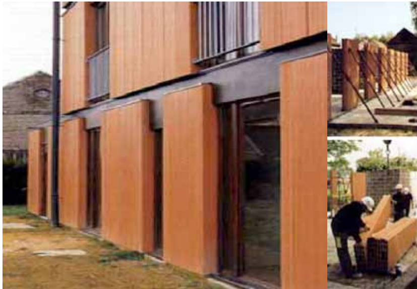
Pic 16- Hotel-management School in Nivillers (F), Tectône, 2000. Construction detail of dry layer facade.
